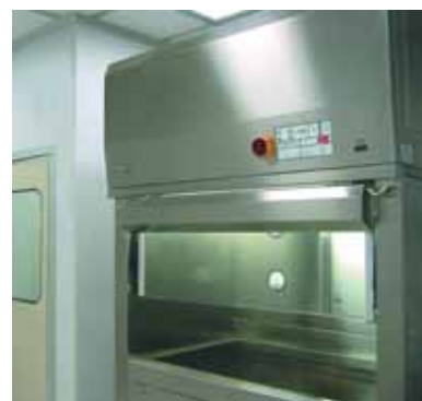
Powder weighing and dispensing cabinet inside a classified environment.
